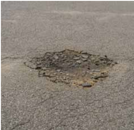
Asphalt Pothole
