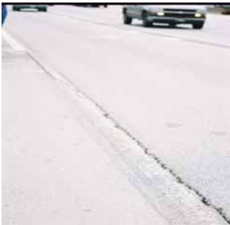
Longitudinal Crack at Edgeline
