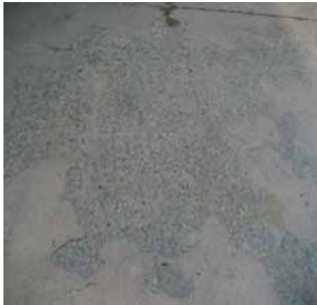
Concrete Scaling
