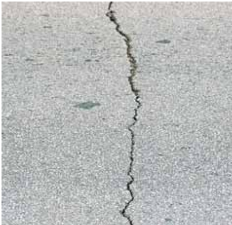
Transverse Crack
