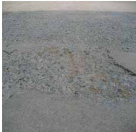
Concrete Scaling
