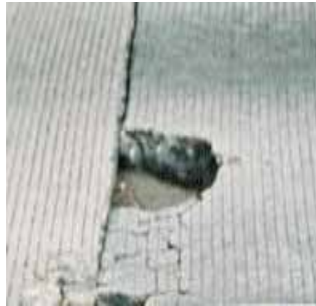
Concrete Pothole
